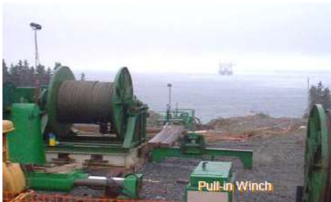
Figure 9-5 Pull-in winch operation
