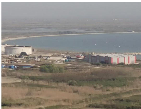
CO2 land-based facilities area
